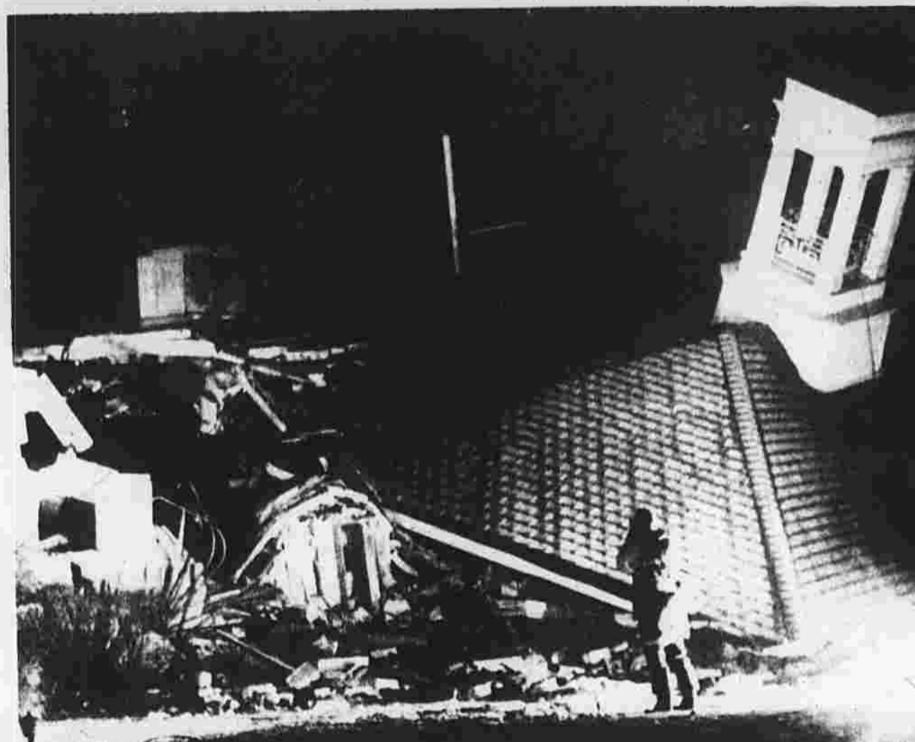
Roof of the two-story Shaker Heights police station rests on the ground after an explosion virtually demolished the building. At least 15 persons were injured. (AP Photofax)
